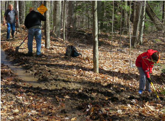
Trenching to Drain Trail
