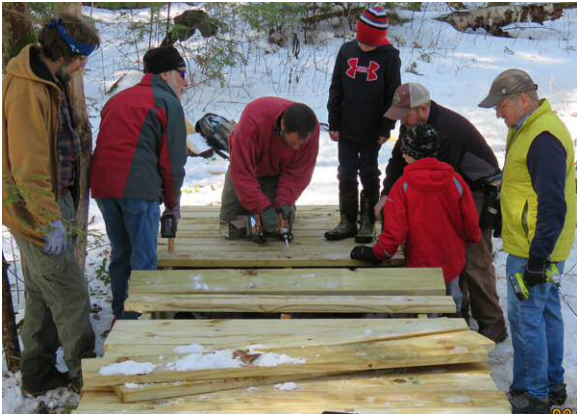
Deck Being Screwed to Stringers
