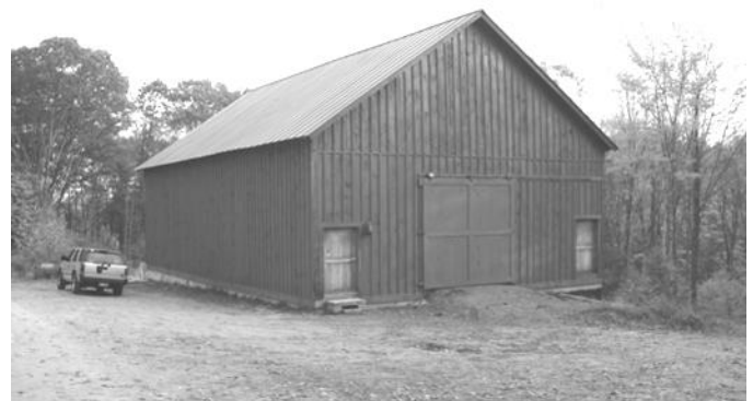
The Barn Paint Job, Nearly Complete
