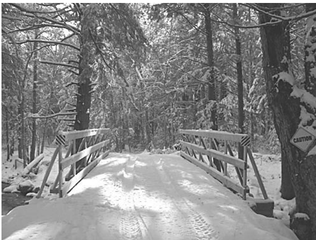
The Rebuilt King's Bridge on Broad Brook Road after the Flood Repairs Were Made
